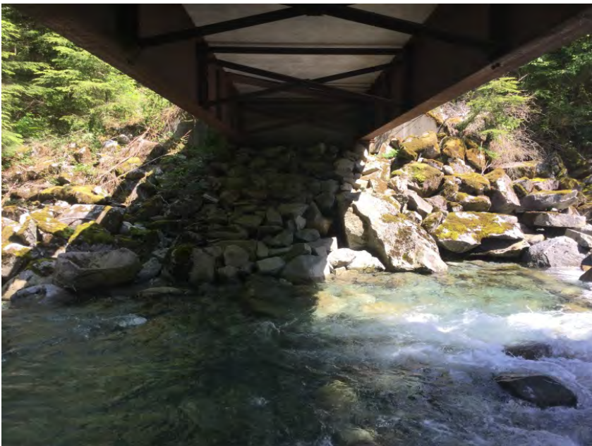
Right Bank Abutment when facing downstream
