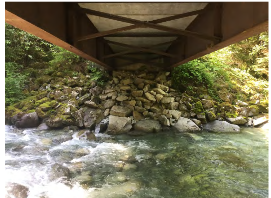
Left Bank Abutment when facing downstream
